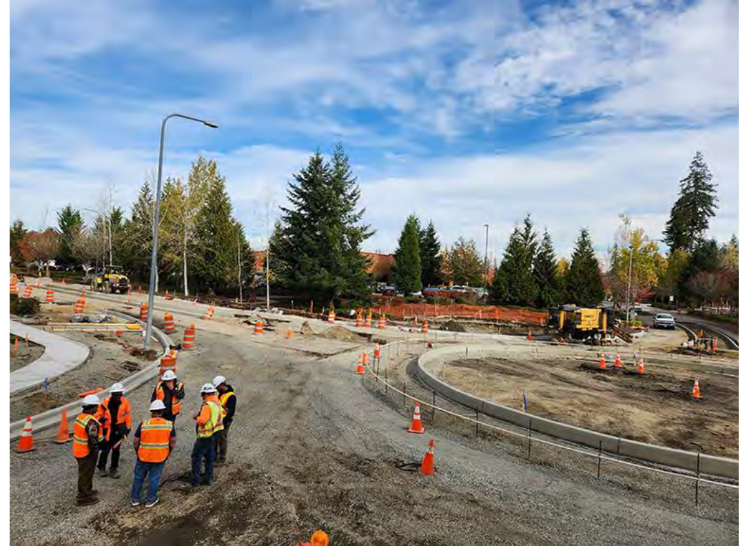
Crews plan the next steps of the Redmond Ridge roundabout at NE Alder Crest Dr.
