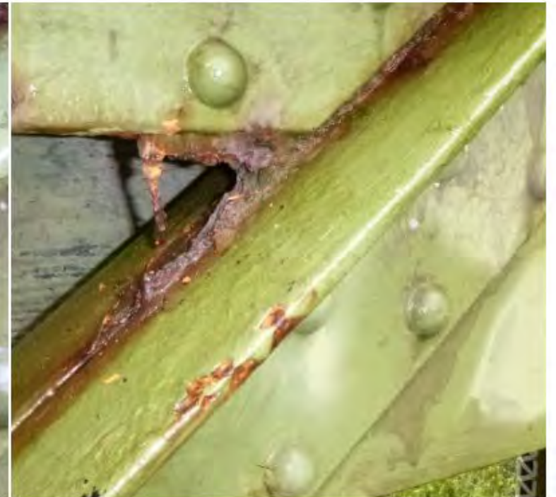
Upper Truss Panel Point 17 East Deck Truss Gusset Plate
