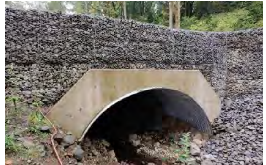
Manley Middle Culvert in Clark County
