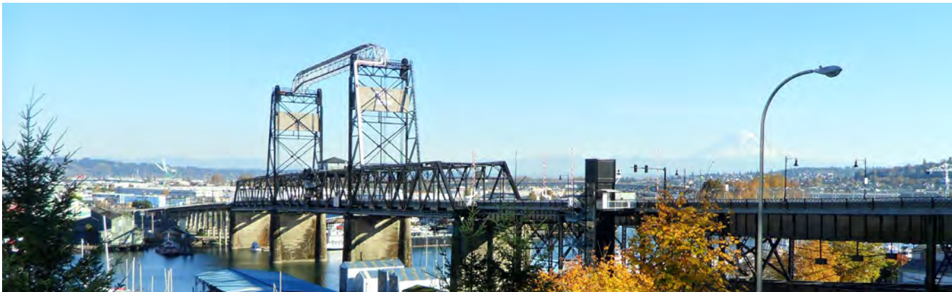
Murray Morgan Bridge in City of Tacoma
