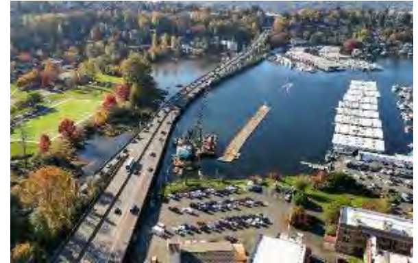
Portage Bay Bridge and Roanoke Lid project
