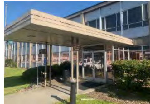
Corson admin building closed November 2024 due to asbestos - 120 staff displaced
