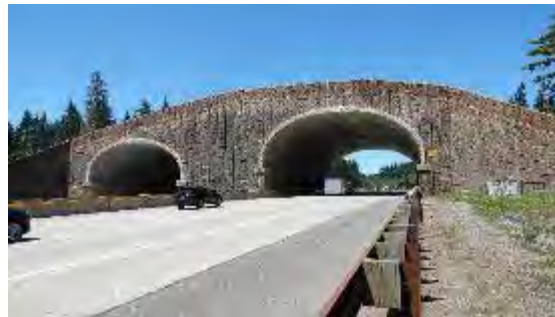
I-90 improvements/ wildlife crossing
