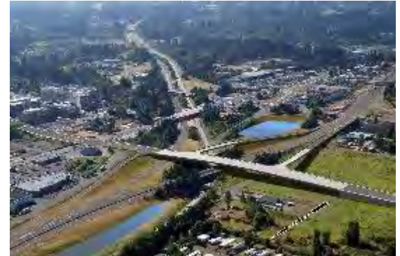
Salmon Creek I-5/I-205 interchange
