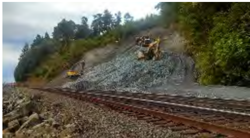
Railroad landslide mitigation, Snohomish County
