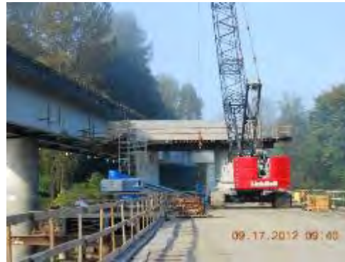
SR 522/Snohomish River Bridge widening
