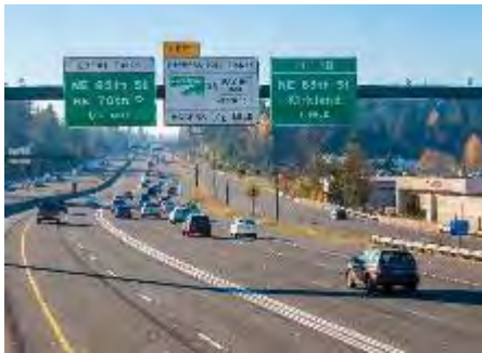
I-405 Express Toll Lanes
