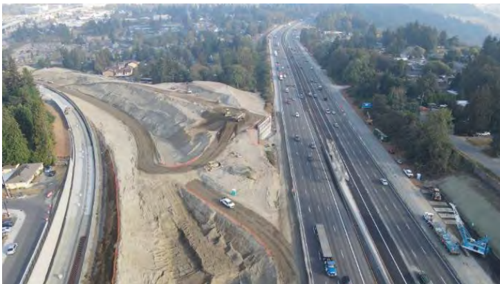
Earthwork along the new SR 509 alignment near I-5
