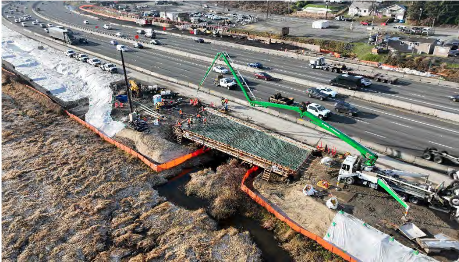
I-5 northbound, pouring new bridge deck
