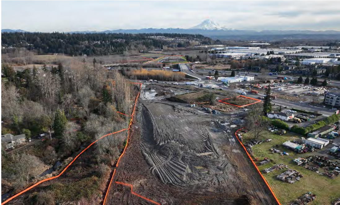
Looking east towards SR 99 roundabout and new Wapato Way East bridge
