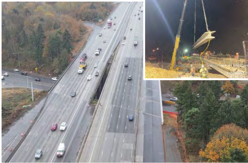
Widening southbound I-5 near the SR 516 interchange
