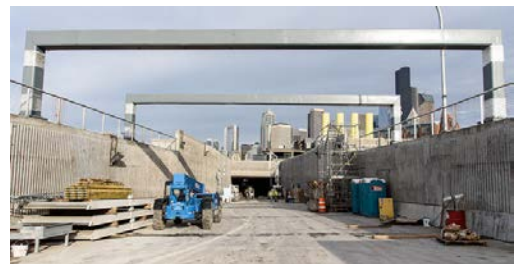
SR 99 Tunnel South Portal – January 2018
