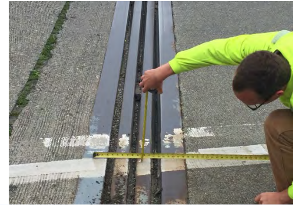
Westbound I-90 Expansion Joint replacement
