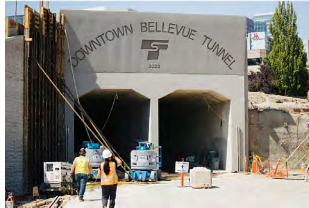
Downtown Bellevue Tunnel
