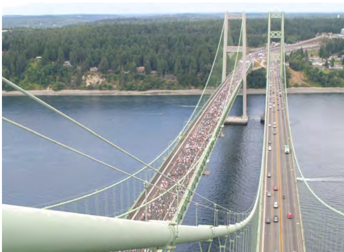
SR 16 Tacoma Narrows Bridge
