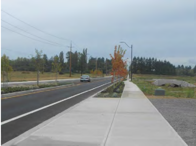
Regional Arterial Upgrades
