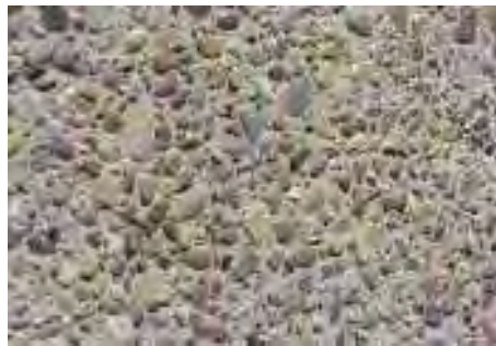
Figure 19: An exposed aggregate surface (Silent Roads, 2003)
