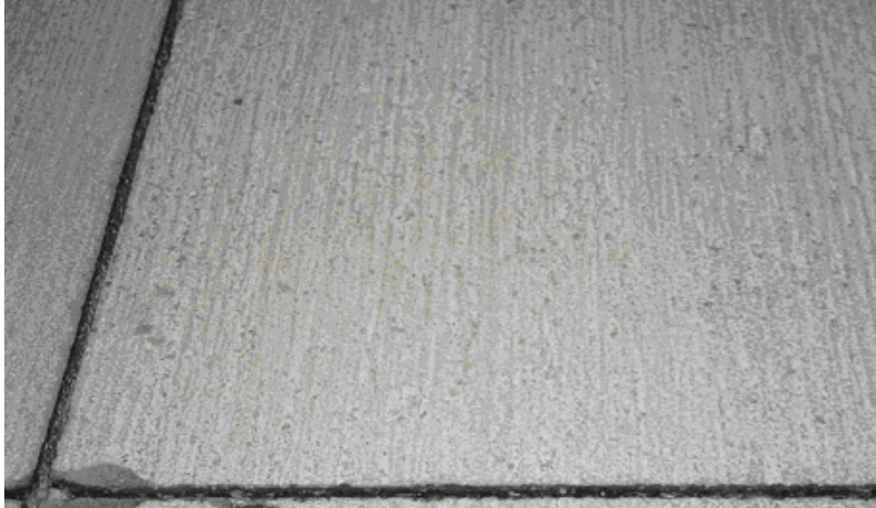
Figure 20: Surface texture from a carpet drag (Anderson et al. 2007).
