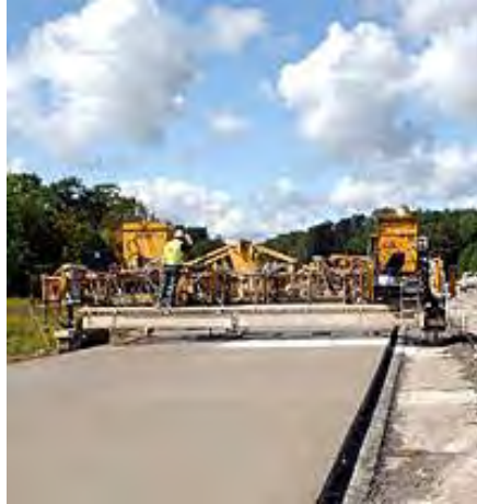
Figure 16: Thin unbonded PCC overlay (Kuennen, 2006)
