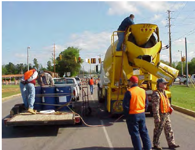
Figure 17: Latex additive going into the grout (Battey & Whittington, 2007)
