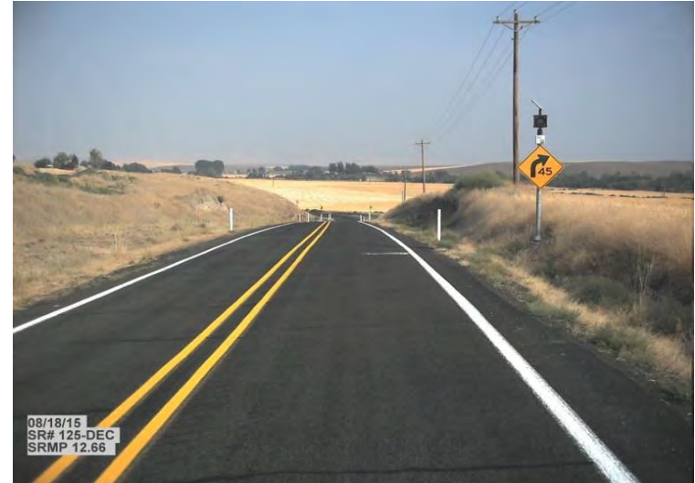
A new flashing beacon in Valley Grove in South Central Region ($6,375)
