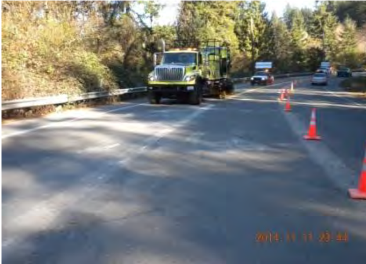
Restriping SR 307 for the closure of Bond Road in Olympic Region, ($4,715)
