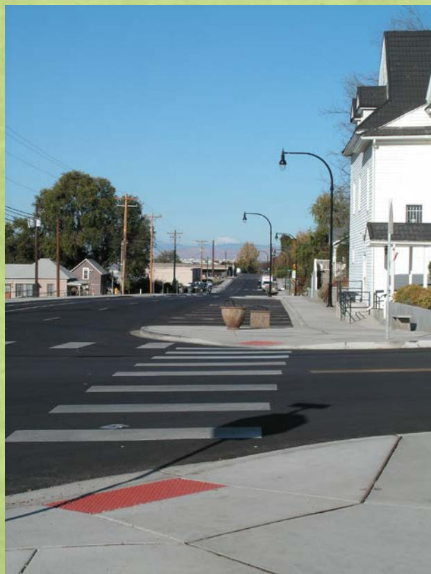
2 nd Avenue and 5 th Street Improvements (2015)
