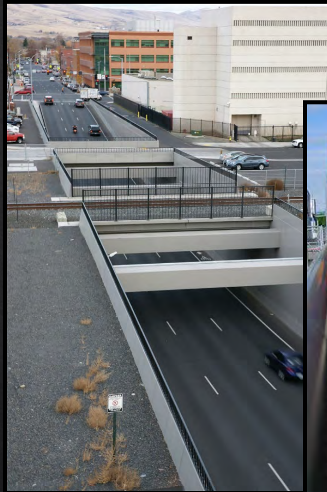
MLK Jr. Blvd underpass (Eastward)
