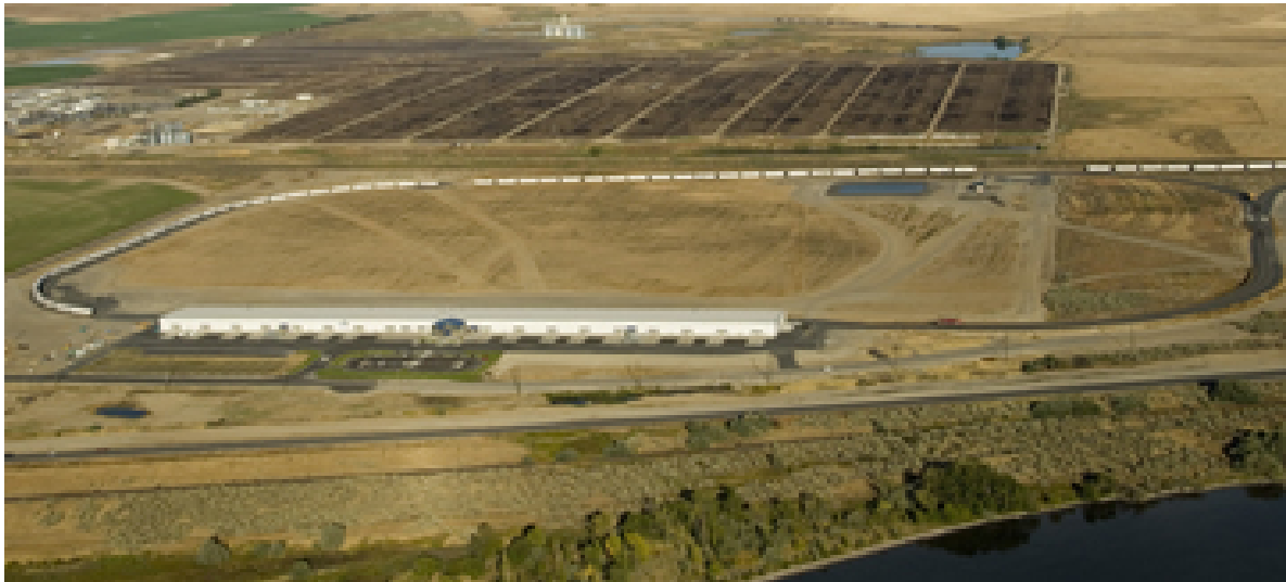
Figure 1. Train Entering the Railex Facility in Walulla, Washington
