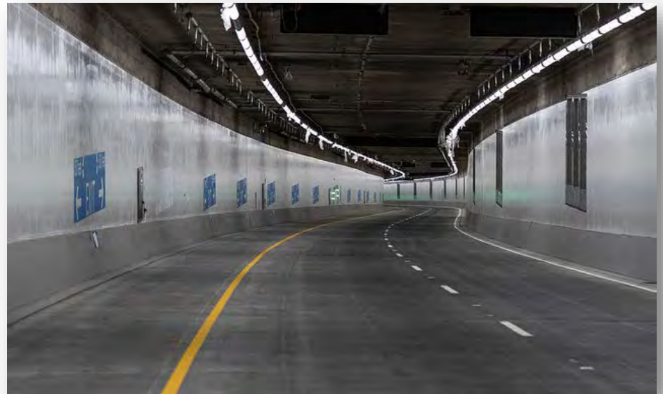
Photo Courtesy WSDOT: Northbound lanes in the SR 99 Tunnel (August 12, 2018)
