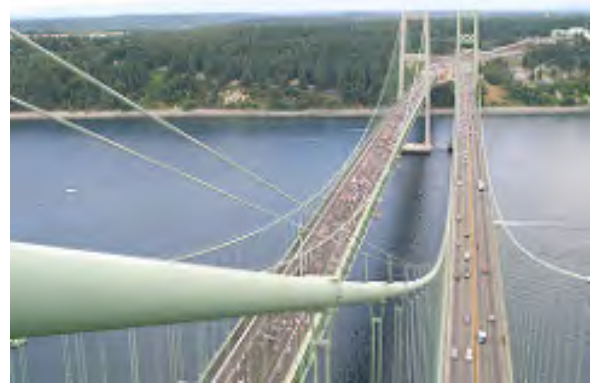
SR 16 Tacoma Narrows Bridge
