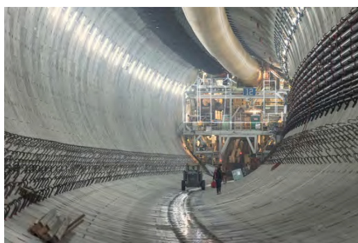
Boring machine in SR 99 tunnel, December 2016
